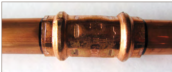
Figure 11.16. Completed installation of a press-connect joint
