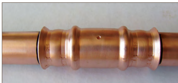
Figure 11.19. Completed joint with insertion marks visible
