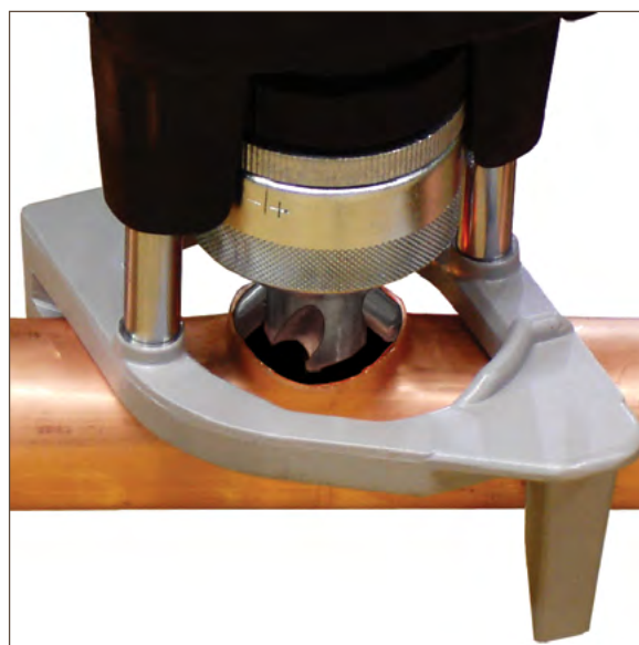
Figure 13.7. Forming the outlet
