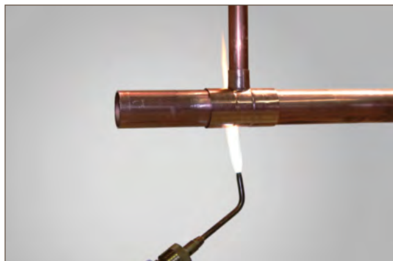
Figure 7.14. Preheating Fitting
