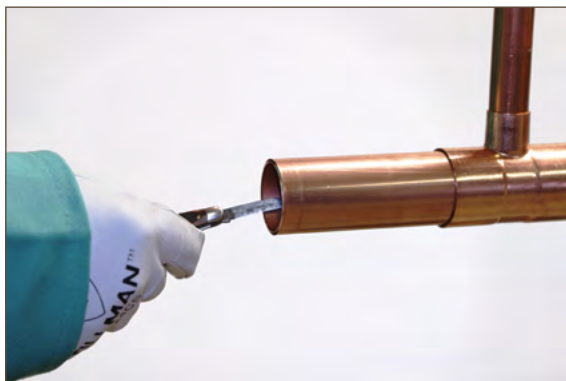
Figure 7.4. Reaming: Pocket Knife
