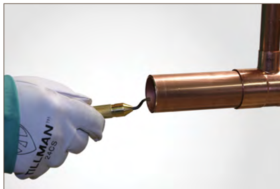
Figure 7.5. Reaming: Deburring Tool
