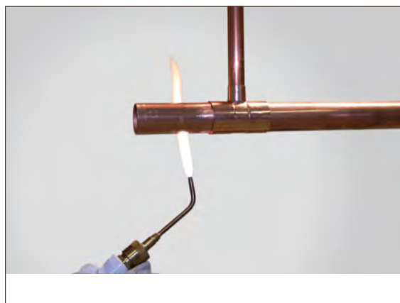
Figure 7.13. Preheating Tube
