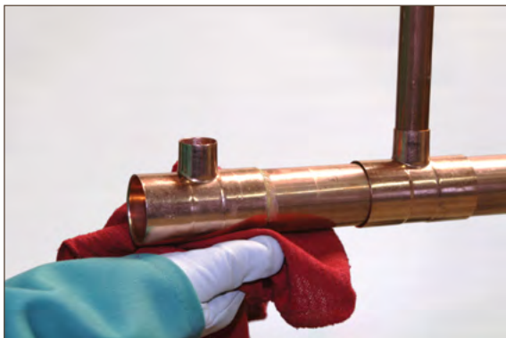
Figure 7.12. Removing Excess Flux
