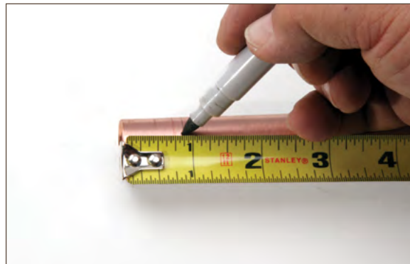
Figure 12.10. Making insertion depth
