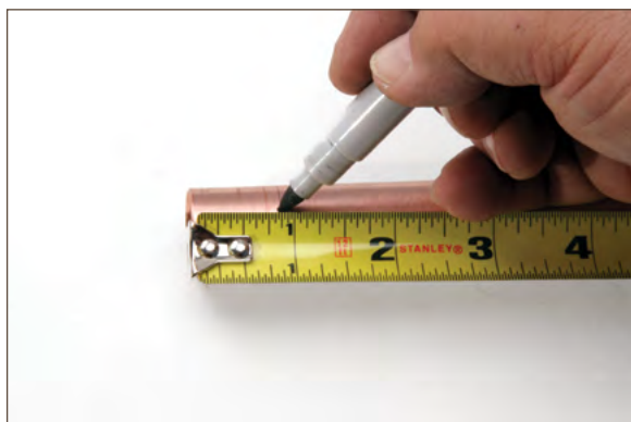
Figure 11.12. Measuring depth of insertion
