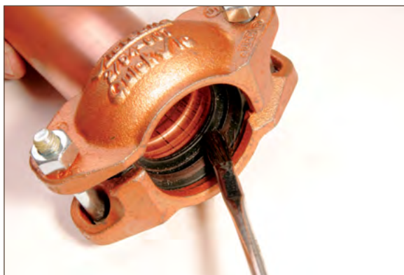
Figure 10.8. Applying lubrication to gasket
