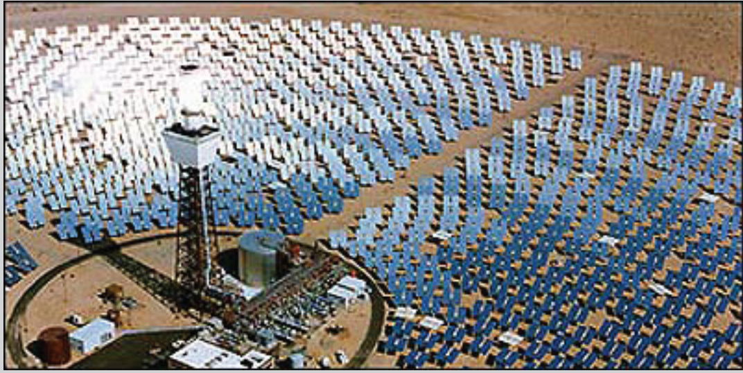
The Solar II power plant near Barstow, CA, used almost 2000 mirrors and the heat of the sun to make 10 megawatts of power.
